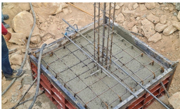
Concrete reinforced with steel bars (rebar)
