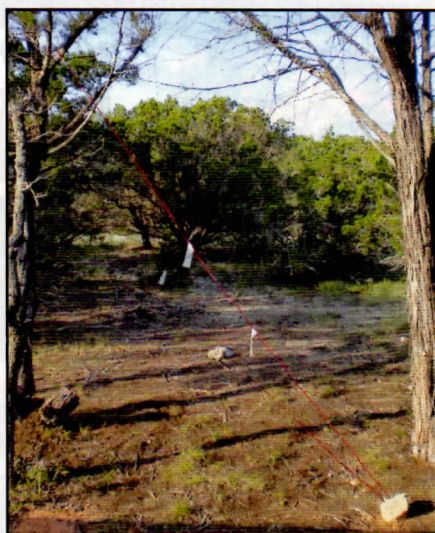
Figure 2 — If the antenna wire were black or gray, it would be even harder to see. Good for an inconspicuous installation. I needed to add the white ribbon so I wouldn't blunder into it while walking around. Note the "high tech" rocks holding the antenna down.
